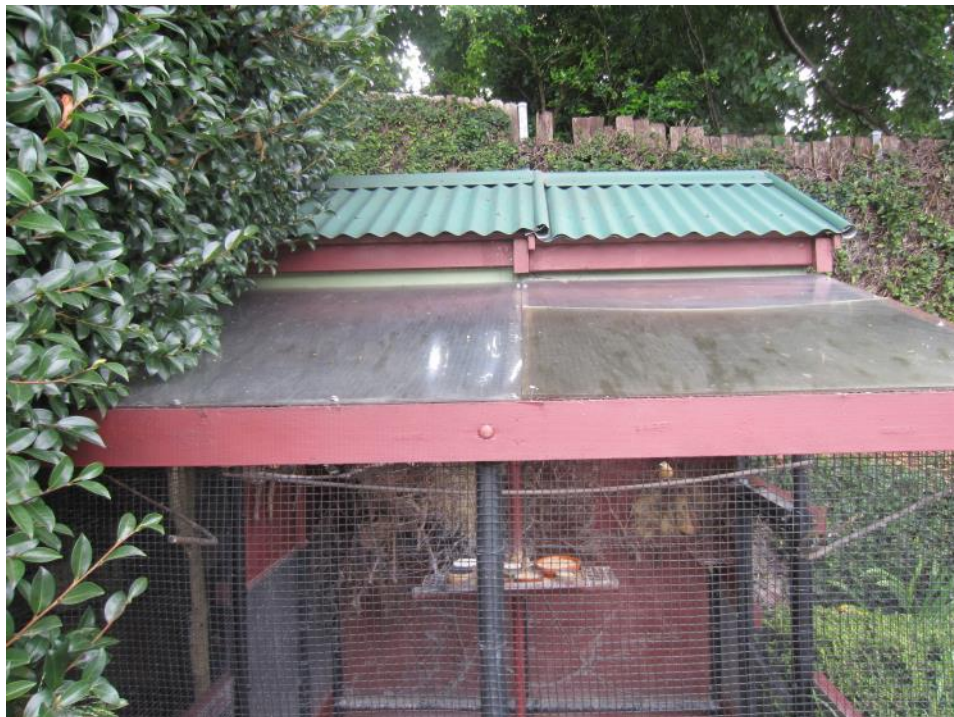
Perspex sheets provide additional protection from wild birds and weather.
